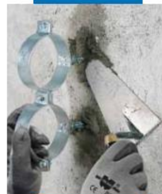
Fixing brackets for pipes using Lamprocem
