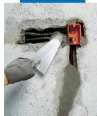
Fixing enclosures and electric cable tubes using Lamprocem
